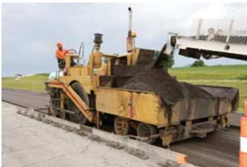
A Blaw-Knox PF220 paved the recycled cold mix.
